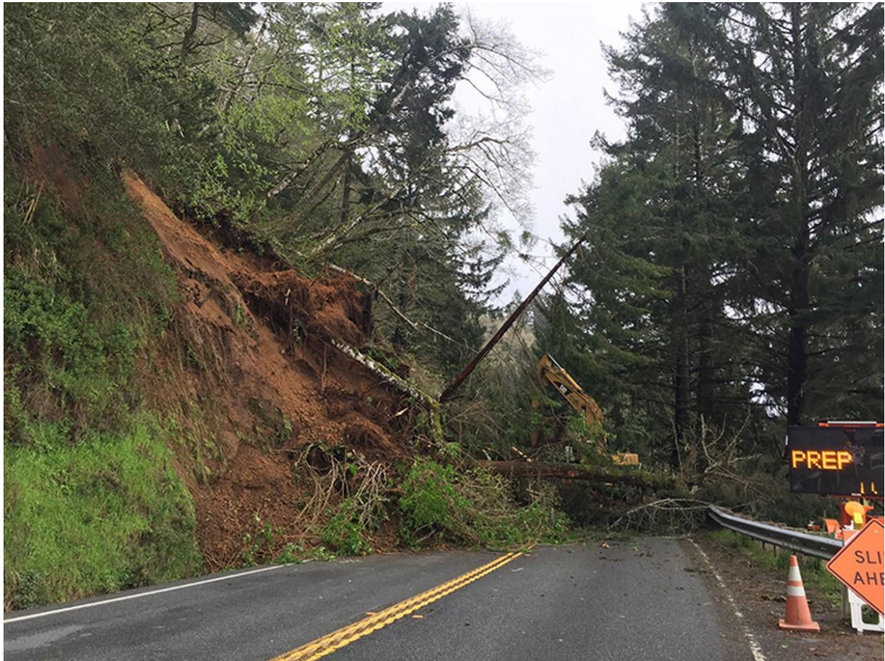
Figure 1 - Last Chance Grade Landslide 1
