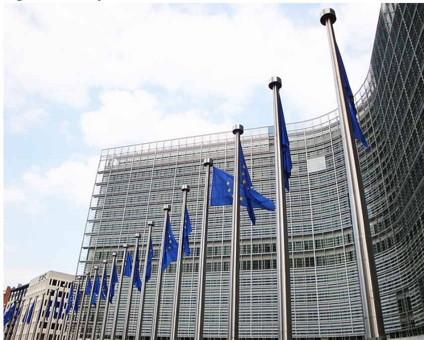
Figure 10 – European Commission Building in Brussels Credit: Jai79 , Creative Commons CC0 1.0 Universal Public Domain Dedication
