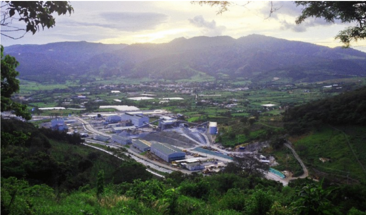
Figure 7 – Aerial View Photograph of the Escobal Mine in San Rafael Las Flores Credit: Tahoe Resources , public domain
