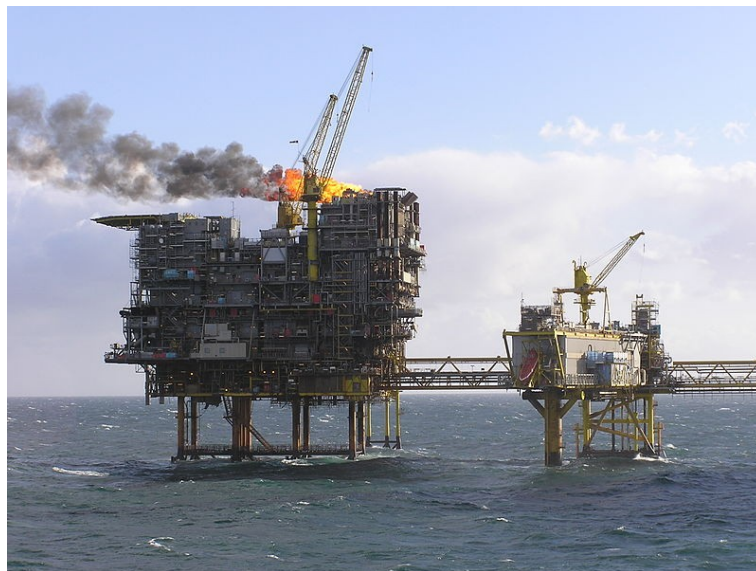
Figure 11 – Tyra East Production Platform ca. 2006 Credit: tom jervis, Creative Commons Attribution 2.0 Generic license
