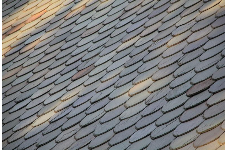
Figure 3 - Slate Roof
