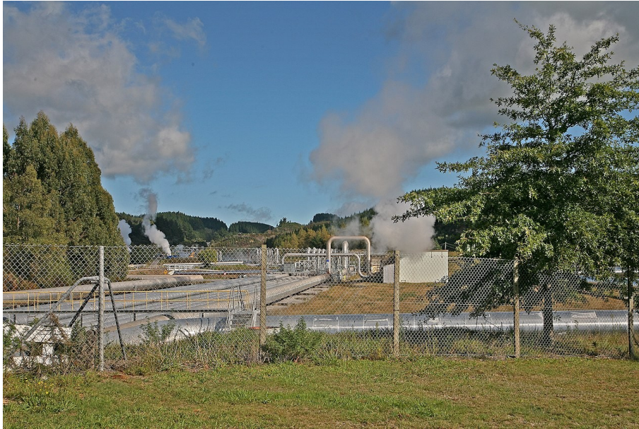
Figure 11 - Wairakei Geothermal Power Plant
